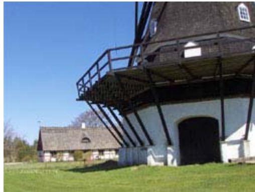
Mill and house
